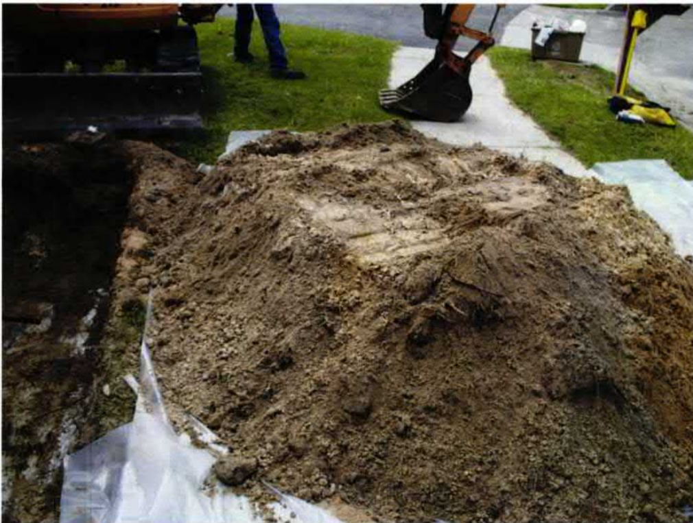
Picture 2: UST 1273 Flamingo excavation in progress.
